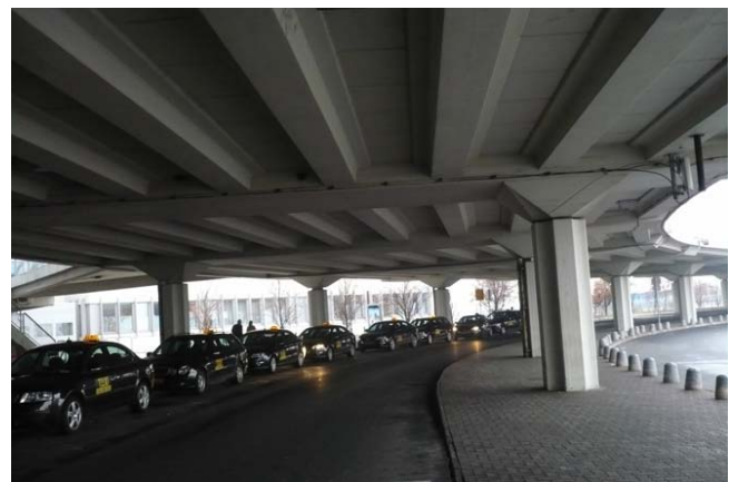
Fig. 7. Covered road in front of the terminals at the Budapest airport
