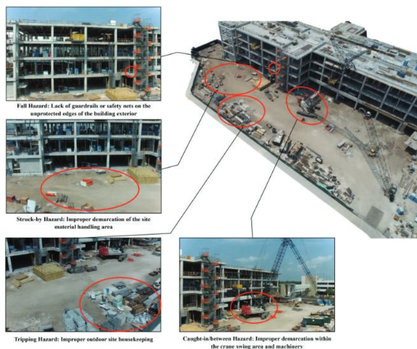
Figure 15. An example of Workplace Safety Inspection with UAS [147].
